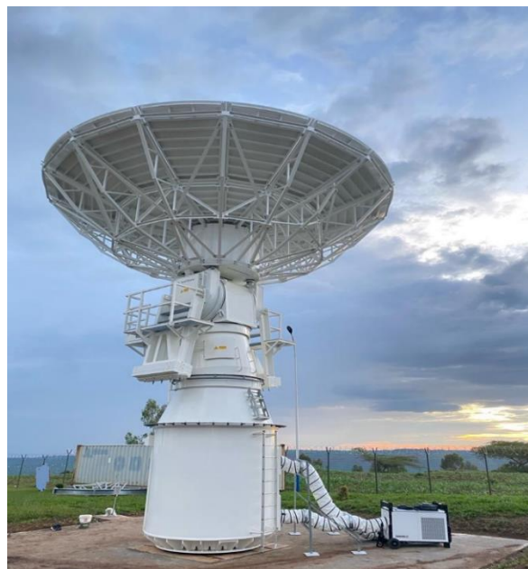
The 9.3m diameter ground station installed at the Teleport Site
